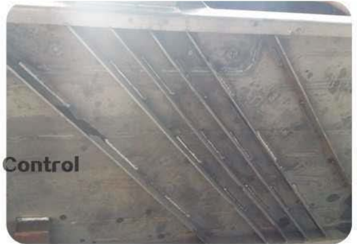
Weld appearance detail on shaker basket
